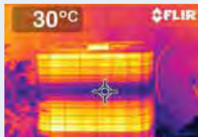
What a thermal imaging camera sees.
