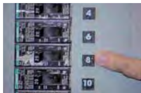
The hotspot indicates a short circuit that can potentially start a fire.
