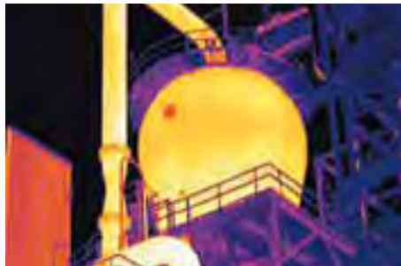
Refractory insulation inspection on a petrochemical reactor
